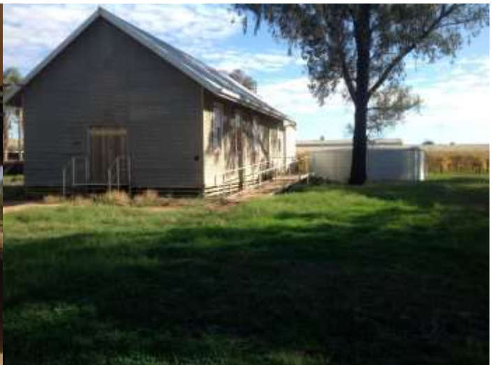
Merbein South Hall (next to Water Storage Tank)
