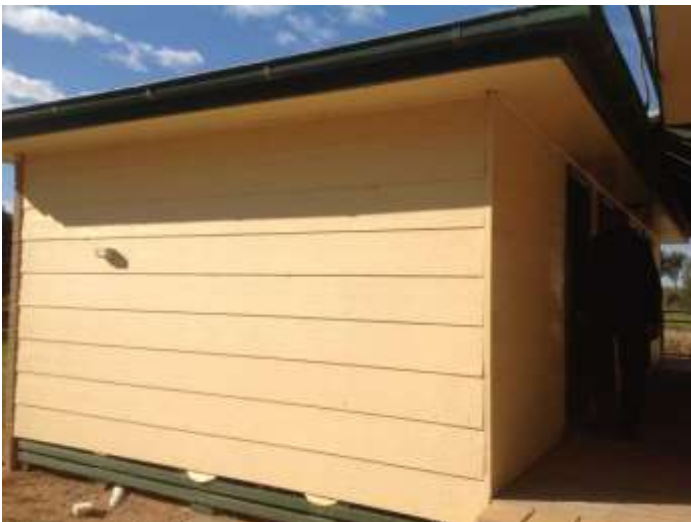
Toilet Block (South Campus)
